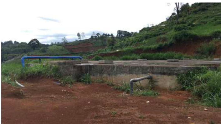
Site Research: Dago Pakar Resor construction site
