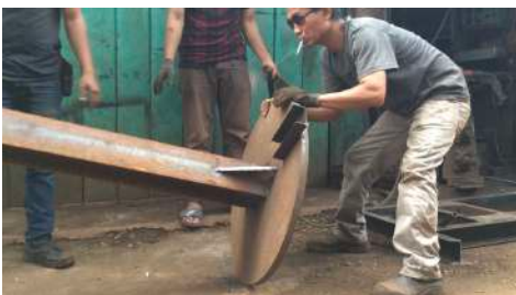
Workers with the H-Beam
